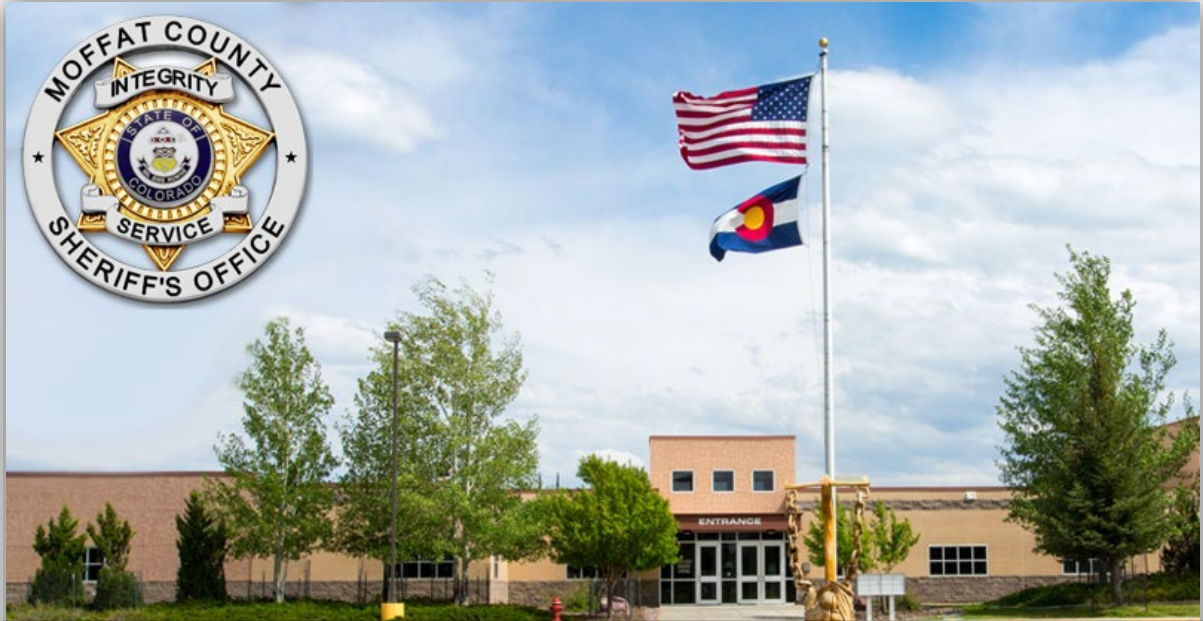
Moffat County Public Safety Center
