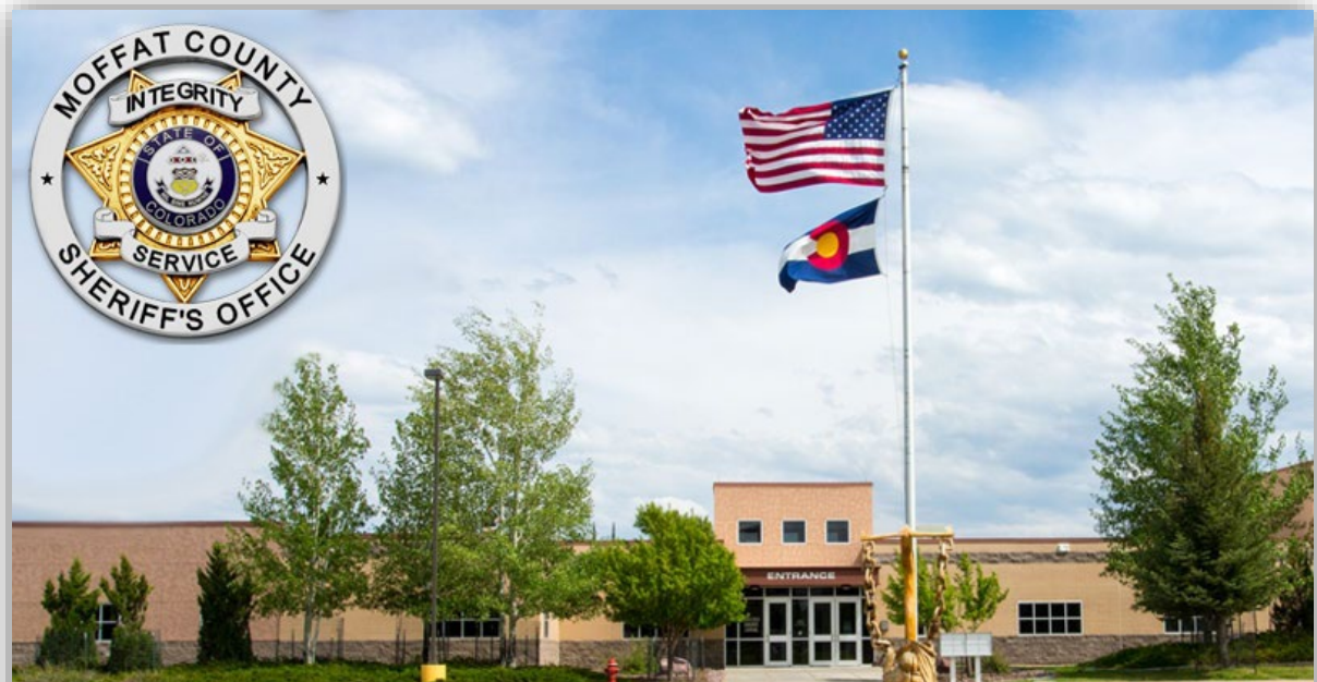
Moffat County Public Safety Center
