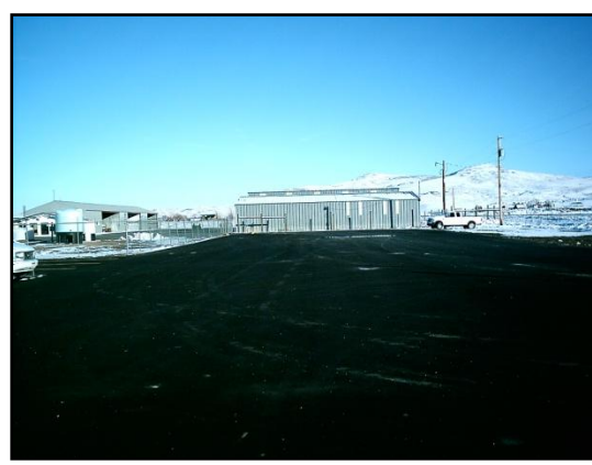
Terminal Parking Lot after Project
