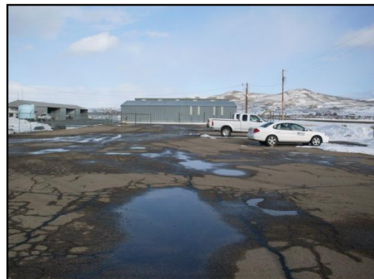
Terminal Parking Lot Prior to Paving
